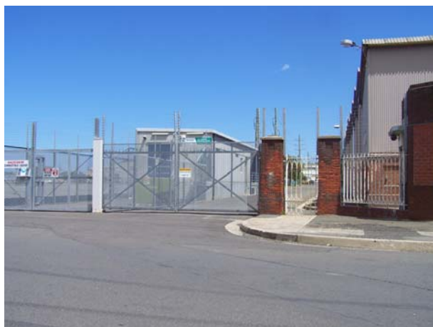
Figure 6: Electrical substation and industrial development adjacent to the western boundary of the subject site and fronting Darcy Rd
