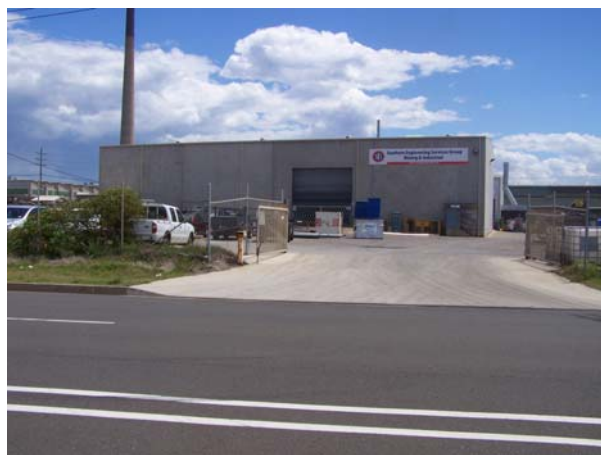
Figure 4: Existing industrial use on southern portion of Lot 103
