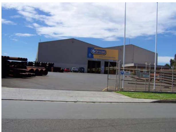
Figure 5: Industrial development on the northern side of Darcy Rd
